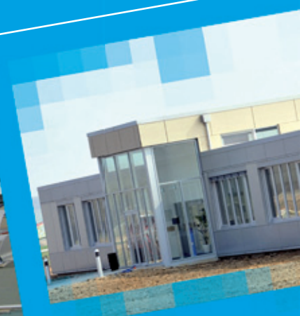
Renewable energies packed in a volume of 543 m 3 : REHAU has used it supplies to the construction of geothermal, Canadian water low-temperature heating panels, obscure double recovery, all in a low-carbon
